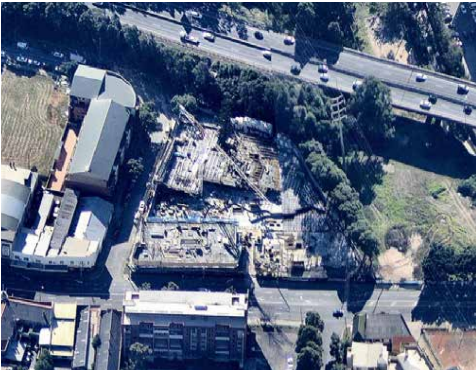
Aerial photograph of site and near context from south showing current Development Application under construction (July 2016)
